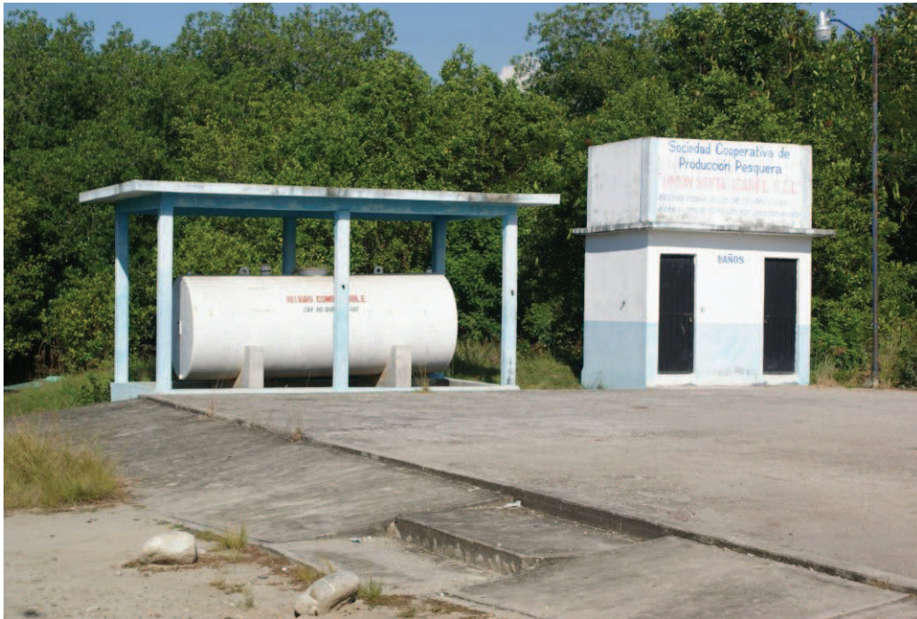
Figure 29: Abandoned infrastructure (fuel tank)
